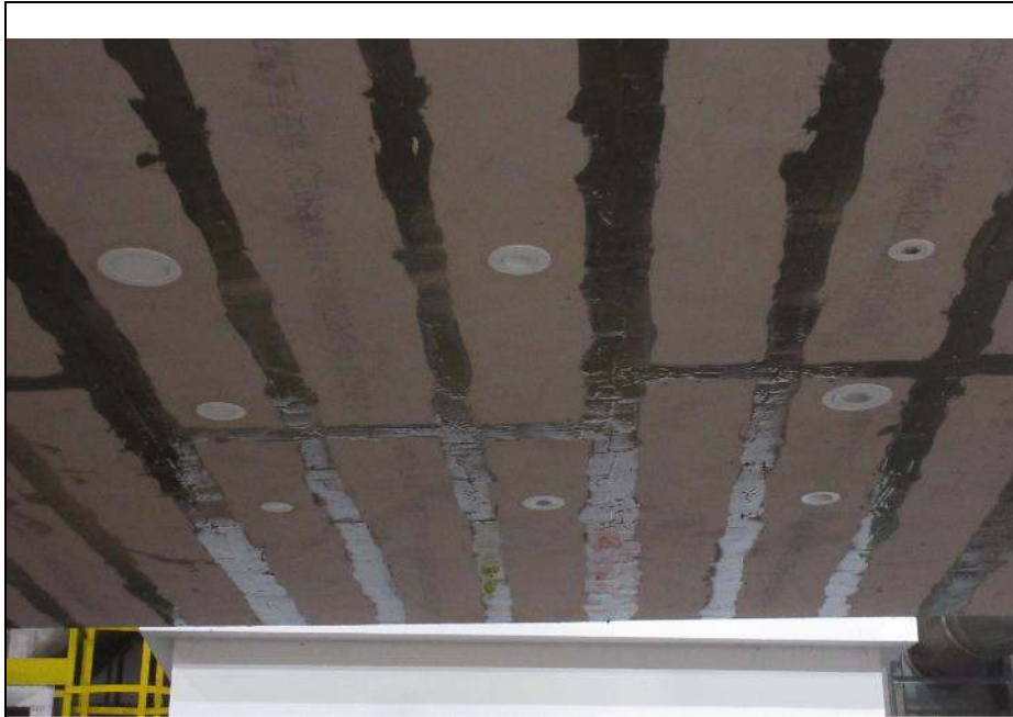
The exposed face before the test
